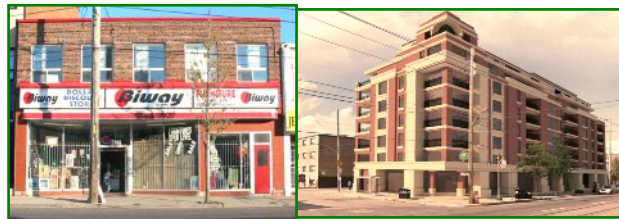
THE BIWAY AND VACANT OFFICE BUILDING NEXT DOOR AT Lake Shore Blvd., and Eight St., may soon end up as an eight-to-nine storey mixed-used condo (right).
