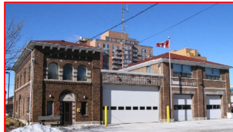
FIRE STATION 435 was built in 1929 to service the growing area.
