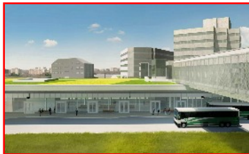
PART OF THE sprawling facility.
