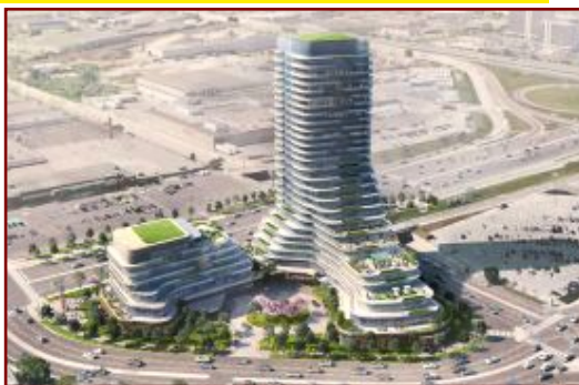
A NEW ETOBICOKE CIVIC Centre, library, gym and health centre are also being constructed.
