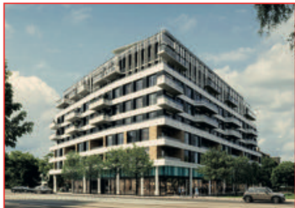
CITY COUNCIL IS CONSIDERING THIS NINE STOREY mixed housing complex proposed at the site of the Mimico strip plaza, at 2491 Lake Shore Blvd. W. at Mimico Avenue, where some businesses are still open.
