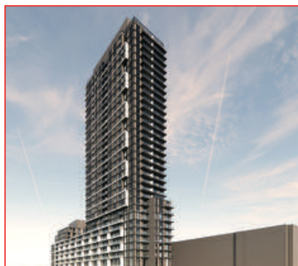
COUNCIL IS ALSO reviewing a proposal to build a 10 storey building, with a 33 storey tower, (above) on a four-block area at 2405 Lake Shore Blvd. W., at Birds and Beans Coffee. Courtesy photos.
