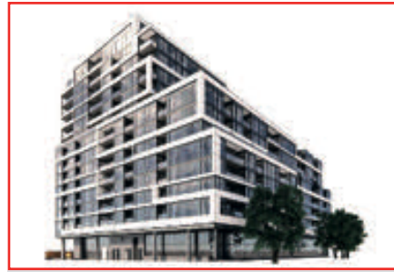
THE 11-STORY 859 THE QUEENSWAY is being built at Plastics Avenue.
