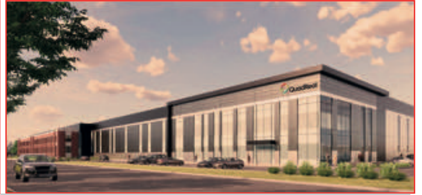
THE NEW CAMPBELL'S facility will be state-of-the-art and user friendly.
