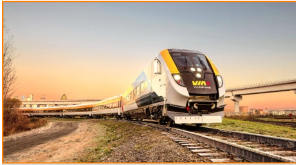
WORK HAS BEGUN ON A Drummond Street maintenance centre (below) to accommodate a new fleet of trains (above and right). Photos by CP rail.
