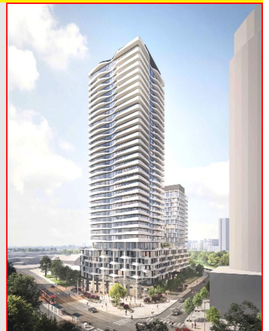
TWO CONDOS ONE AT 35 STORIES and the other at 18 stories are being built at a former self-storage site at Lake Shore Blvd., W. and Legion Road. Courtesy photos.
