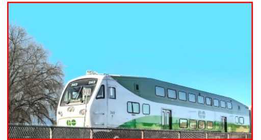
ALSO BEING BUILT at the site are hubs for GO Transit and the TTC.
