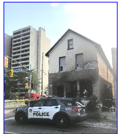
COLIN'S DUGOUT and some of the smoke damage from the fire.
