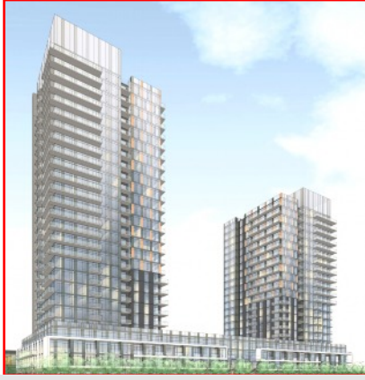
NEW CONDOS at 1061 The Queensway, at Islington Ave., will have a new Longo's and Sobeys.
