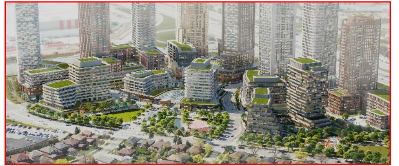
CLOVERDALE MALL when completed (above) will also have two parks and underground parking. The mall as it will look inside (bottom). Photos courtesy of Quadreal Property Group.
