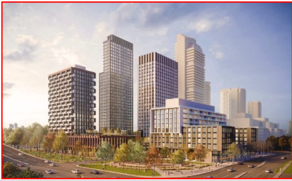
THE FEDERAL GOVERNMENT plans to build 494 rental units at 300 The East Mall.
