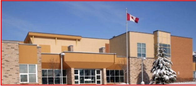
NEW SCHOOL LIKE this one is being built in Central Etobicoke on the site of the Etobicoke Secondary Alternative School (below) which will be demolished.
