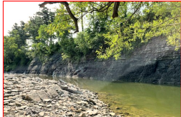
DAMAGE TO ETOBICOKE Creek after last month's storm that washed out pathways. Repairs have been done in areas.
