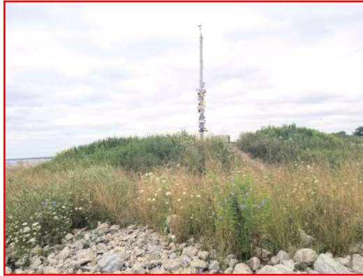
THE LENGTHY WORK will address erosion hazards impacting the park and enhance protection around the shoreline to prevent future hazards to visitors. Birds and wildlife are also protected.
