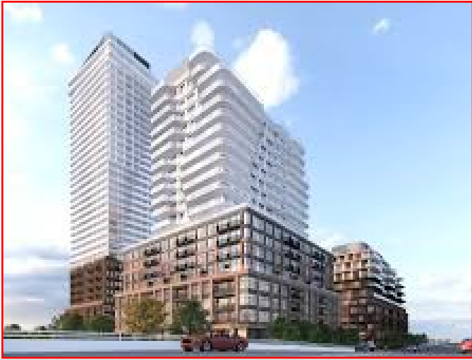
PLANS ARE UNDERWAY for a quiet residential area of Royal York Road at Queen Elizabeth Blvd., to build a 35 and 17 storey condo towers. (above, right).
