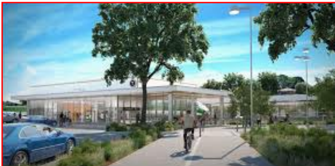
VIEW OF LONG BRANCH GO Station on which work is underway leaving a busy, congested facility with train activity (right).
