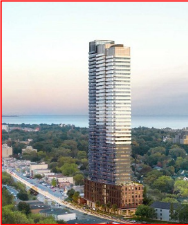
THIS 43-STOREY condo is planned for 3807-3829 Lake Shore Blvd. W., across from the Long Branch GO Station.
