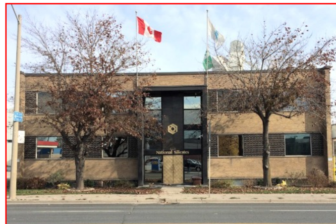
NATIONAL SILICATES IN its heyday employed about 100 employees at this South Etobicoke plant and about 1,500 workers in total across five continents.
