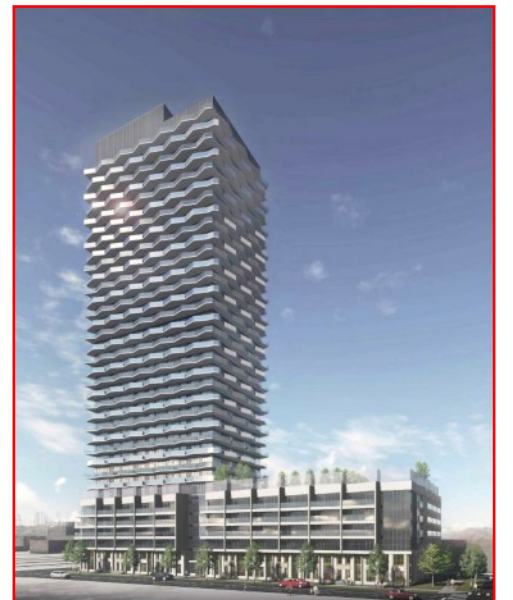
ANOTHER 35 FLOOR tower is under construction at 36 Zorra Street, where a number of buildings are being built. There are traffic congestion concerns once the buildings are completed and people move in.
