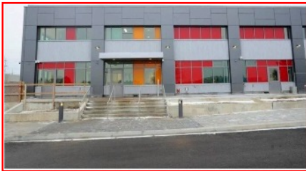
THIS IS what the Third Street shelter will look like when completed in 2030.
