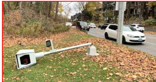
THIS POLE MOUNTED camera at Parkside Drive has been cut down three times.
