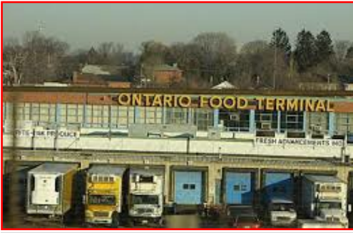
THE ONTARIO FOOD Terminal and below are condos planned next door to traffic and noise concerns.
