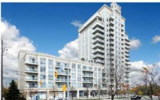
1109-3865 LakeShore Blvd W Tor 2 BR condo with balcony & 1 underground parking. $689,000
