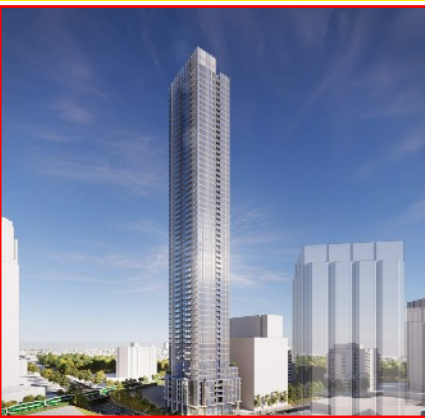
A MASSIVE 61-storey tower, (top, center) planned for near the Islington Subway.
