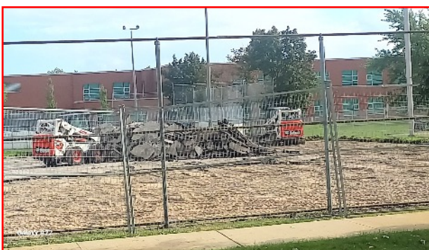
SIR ADAM BECK park being dug up by City crews to install new pickleball courts. Staff photo.
